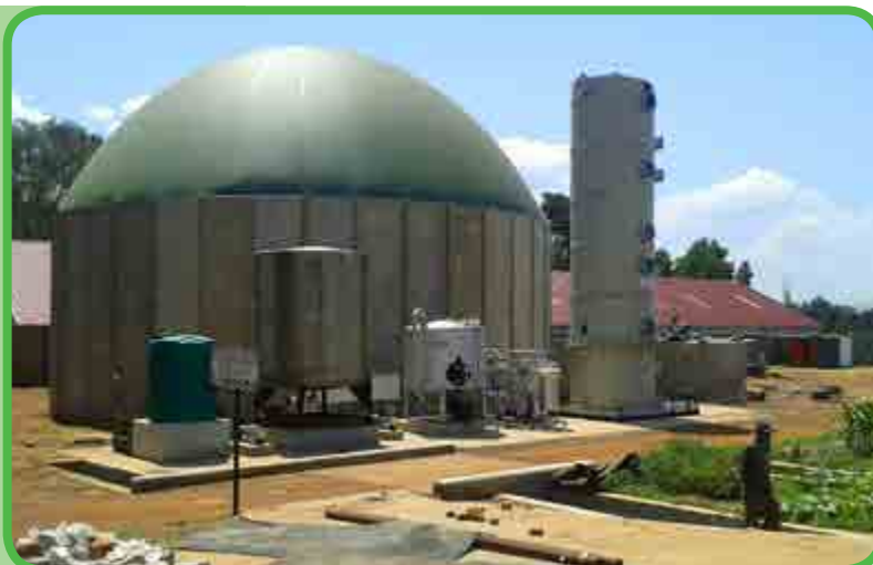
Figure 18: Morgan Springs Biogas Plant (BiogasSA, 2015)
