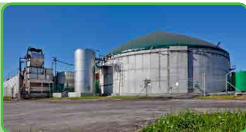
Figure 16: Elgin Fruit Juice Biogas Plant (Energy, 2015)
