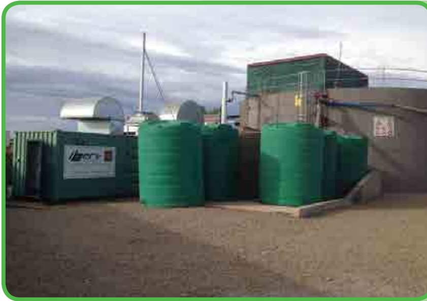
Figure 19: Jan Kempdorp Biogas Plant (iBert, 2015)
