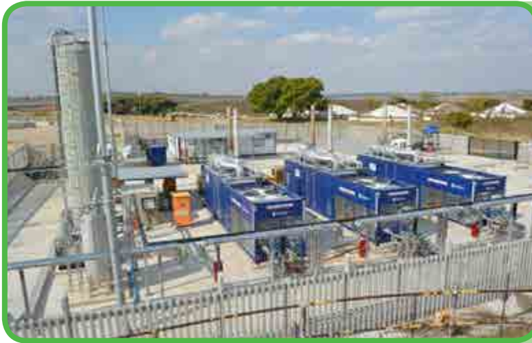
Figure 17: Northern Waste Water Treatment Works (Scholtz, 2013)
