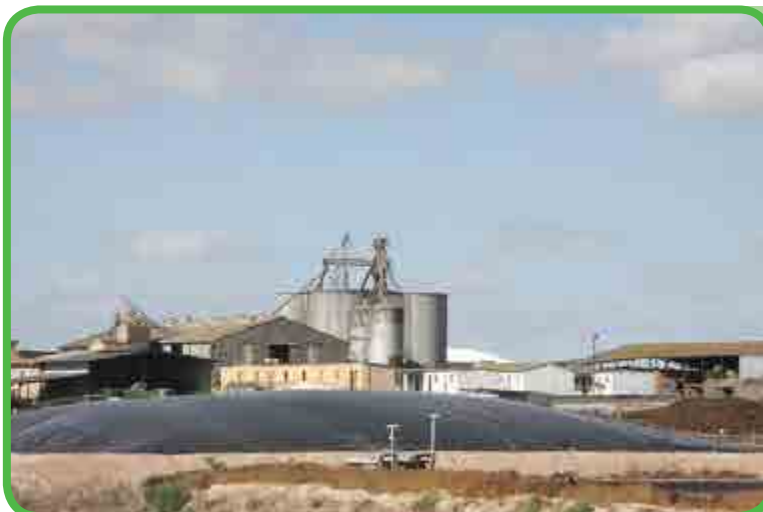
Figure 15: Uilenkraal Biogas Plant (Construction Review, 2015)
